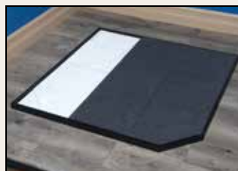
15. Lay in (1) 12" x 36" Modular Panel.
