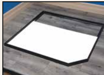
7. Lay in (1) 12" x 36" Micore 300 rectangle piece.
