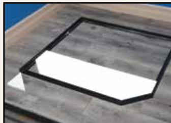
6. Lay in the Micore 300 triangle piece.
